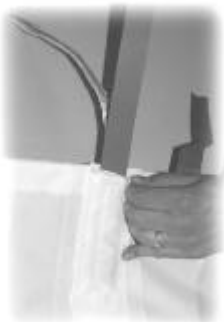
Fitting batten with velcro closure - stage one
