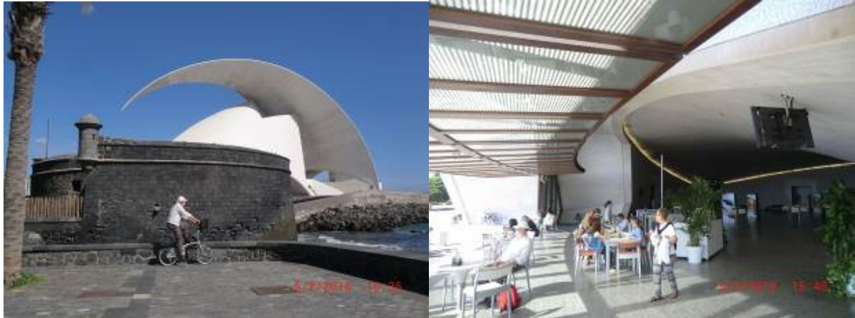
The restored fort, in the background part of the auditorium of Calatrava. The auditorium's entire glass paneled side-wall flips up, creating an immense, shaded terrace. To our surprise a pint of beer (tanque or jara) costed only 3 Euros on this high-class spot!
